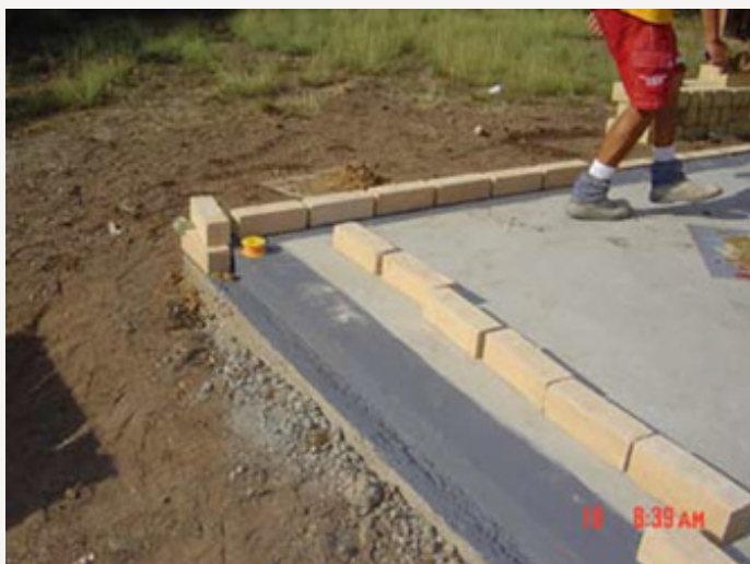
Term Seal and dampcourse coating being applied prior to laying Timbercrete bricks
