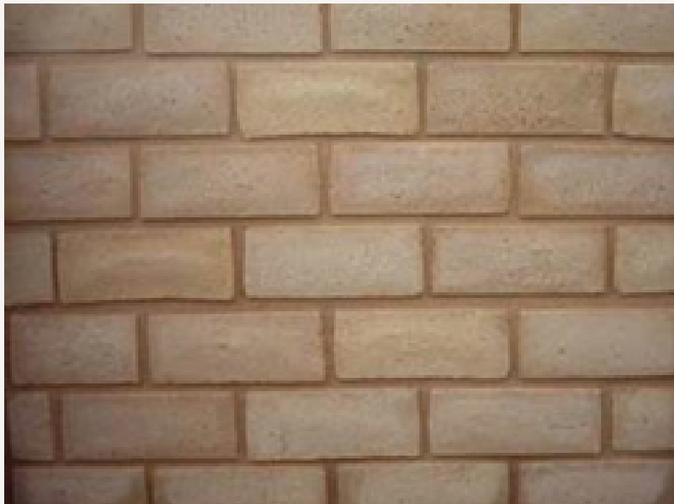
Correct laying of Timbercrete
