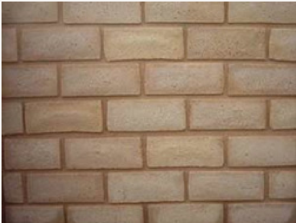
Correct laying of Timbercrete
